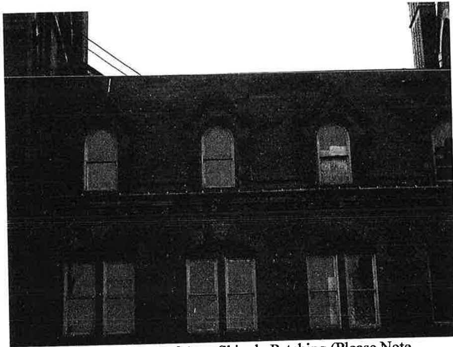
3. Typical Mansard Roof Area Shingle Patching (Please Note Dark Black Areas)
