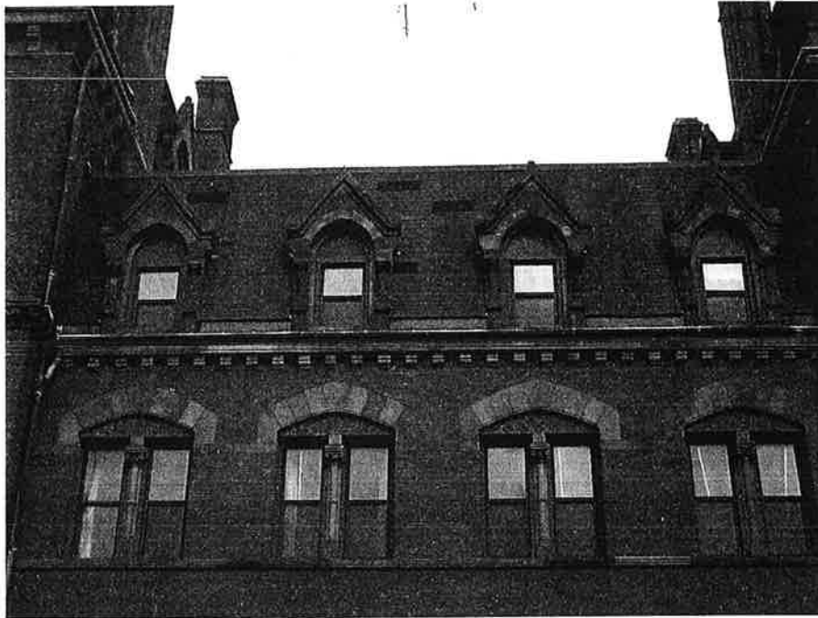
1. Typical Mansard Roof Area Shingle Patching (Please Note Dark Black Areas)
