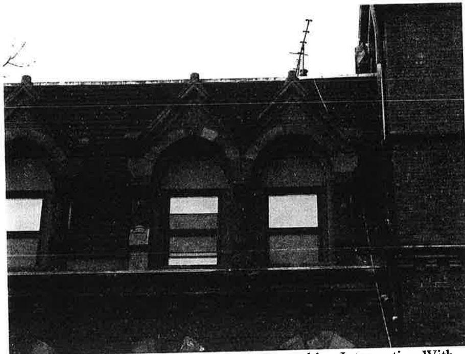
4. Typical Mansard Roof Area Shingle Patching Intersection With Flat Roof (Please Note Dark Black Area)
