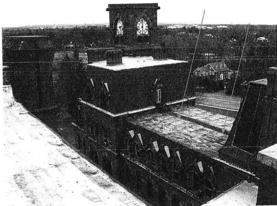
8. Roof Area 11 Mid-Section North-To-South Split Temporary Repair
