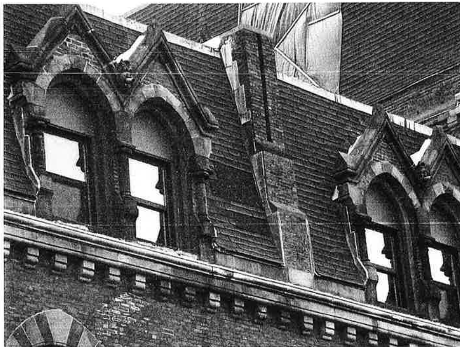
2. Typical Mansard Roof Area: Missing Shingle Patching & Caulking Of Step Flashing Reglets
