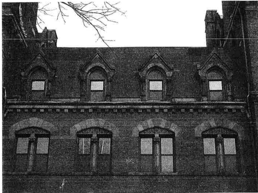
17. Mansard Roof Level Dormers: Typical Single Gable/Single Window Dormers Overview & Details
