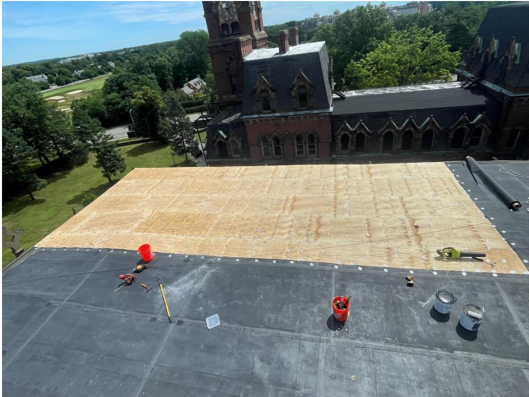
New 1/2" CDX plywood mechanically fastened
