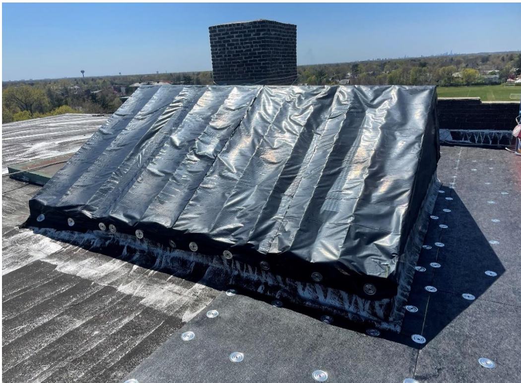
Waterproof existing skylight with membrane
