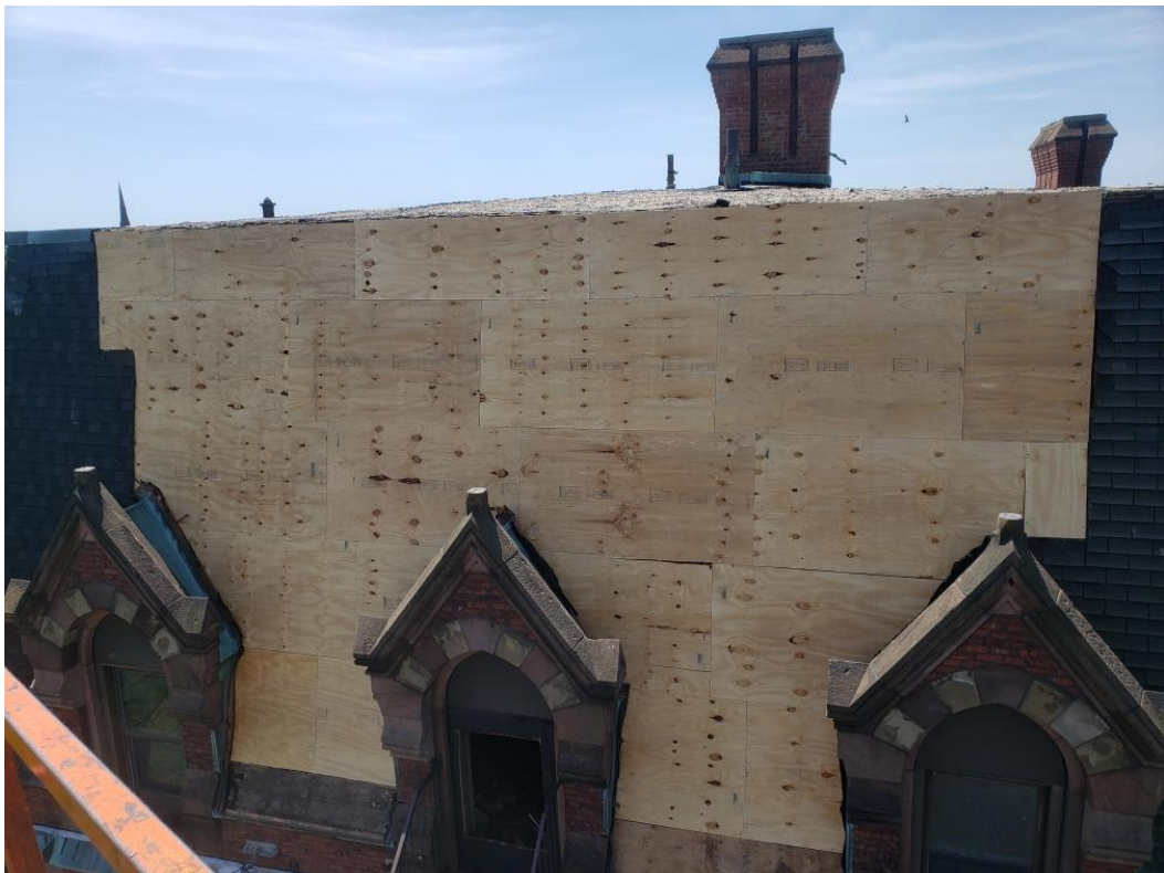
New \frac{3}{4} " CDX plywood sheathing
