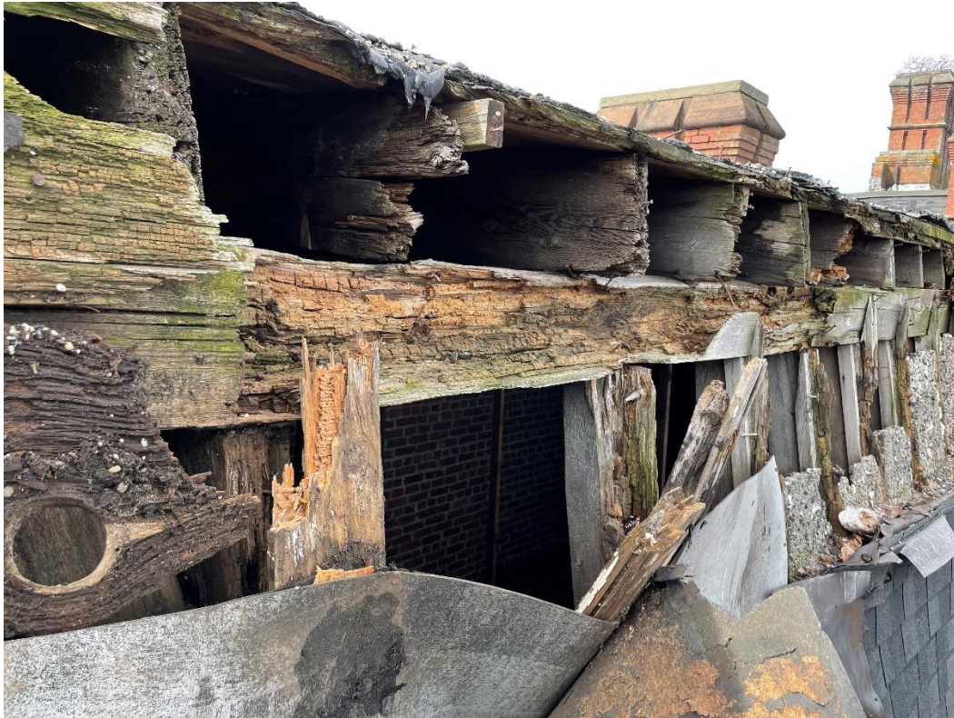
Deteriorated wood structural membrane, (rafters and header beams)
