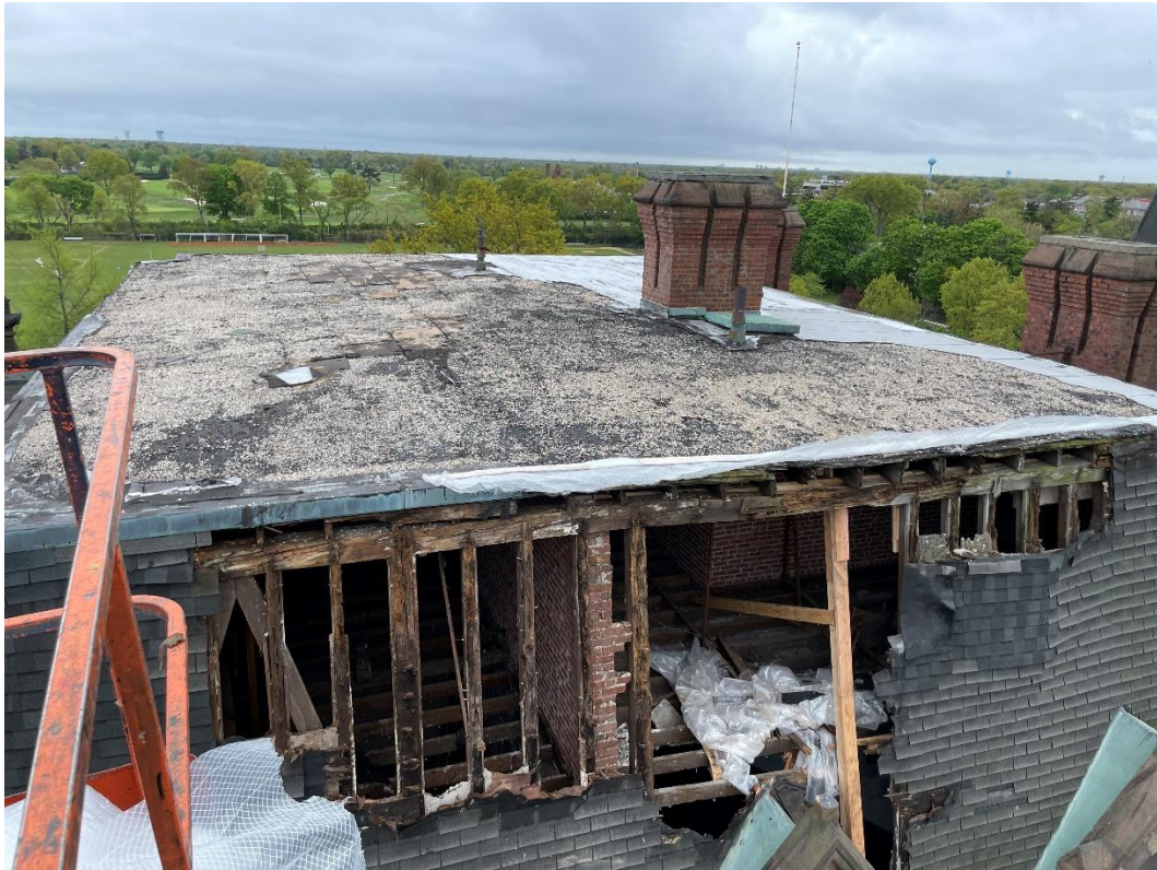
Selective mansard removal and temporary shoring
