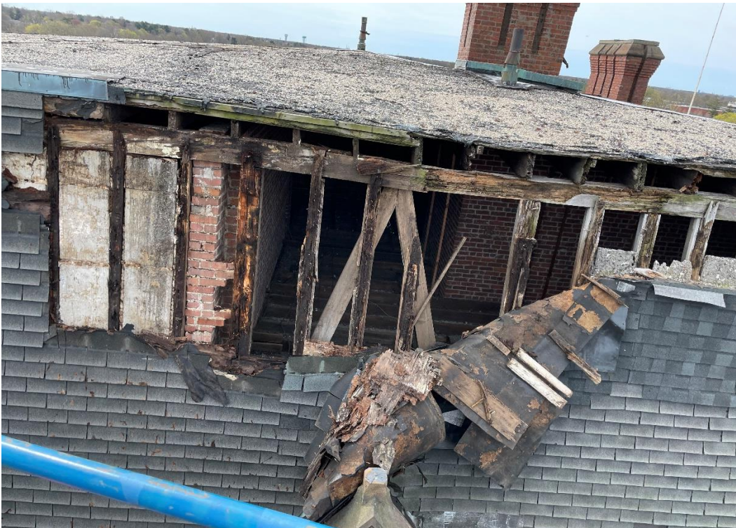
Selective mansard roof demolition
