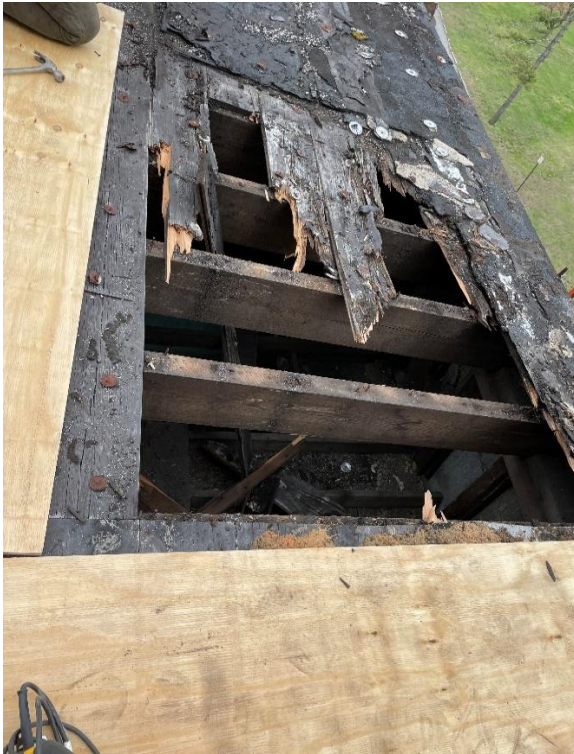
Roof deck patching (Southeast Section)
