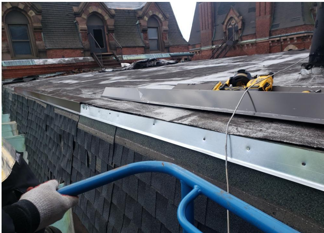
Typical Aluminum Edge Flashing with Cleat
