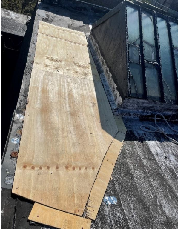
Roof deck patching with plywood
