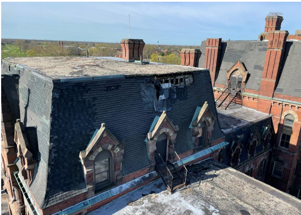
Existing mansard roof conditions, North elevation
