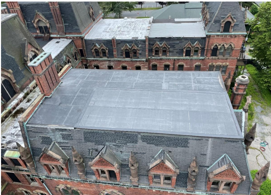
Post Construction: Approximately 900 square feet of EPDM Roofing
