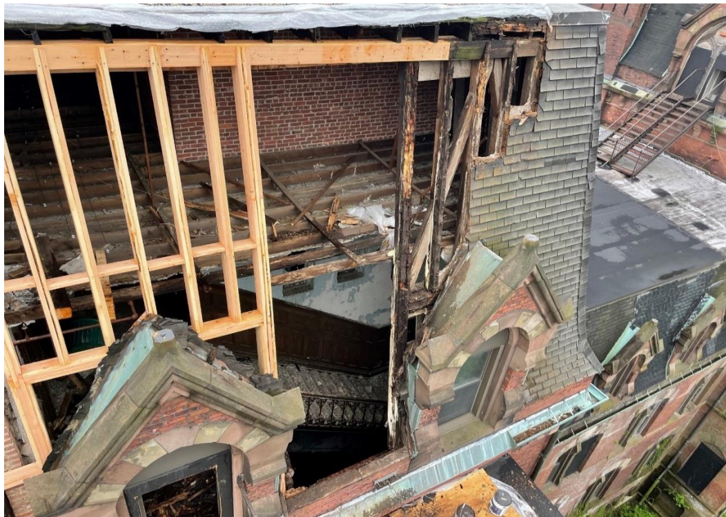
New wood double 2 x 8 rafters & header beam
