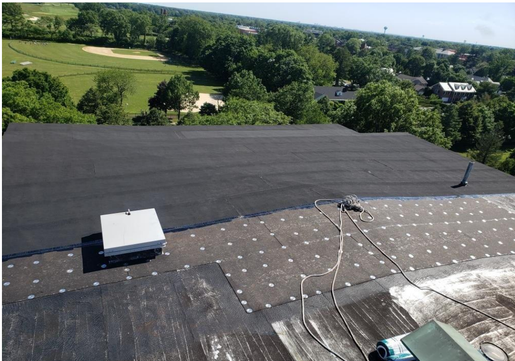
Polyglass One-Ply Roof System Components, (SBS Elastomeric roof membrane over asphalt coverboard)
