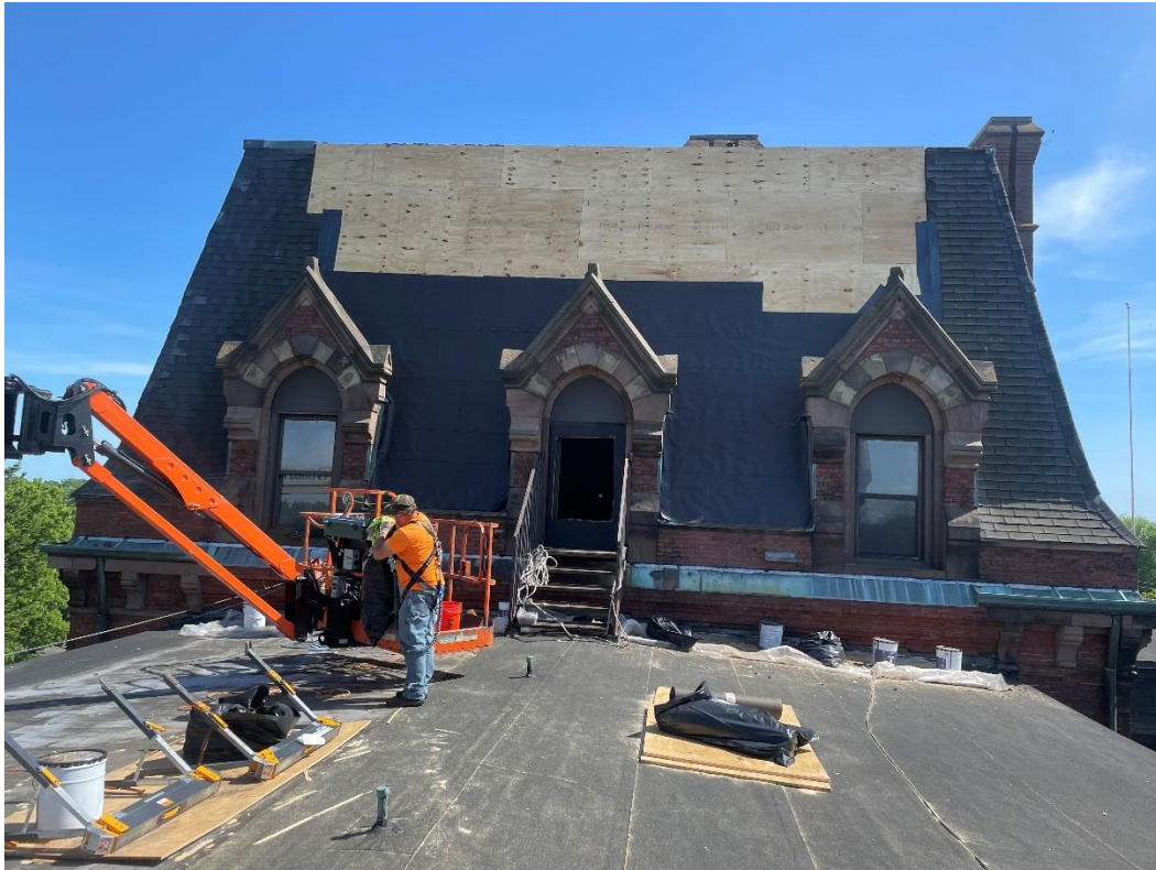
Installation of asphalt saturated felt
