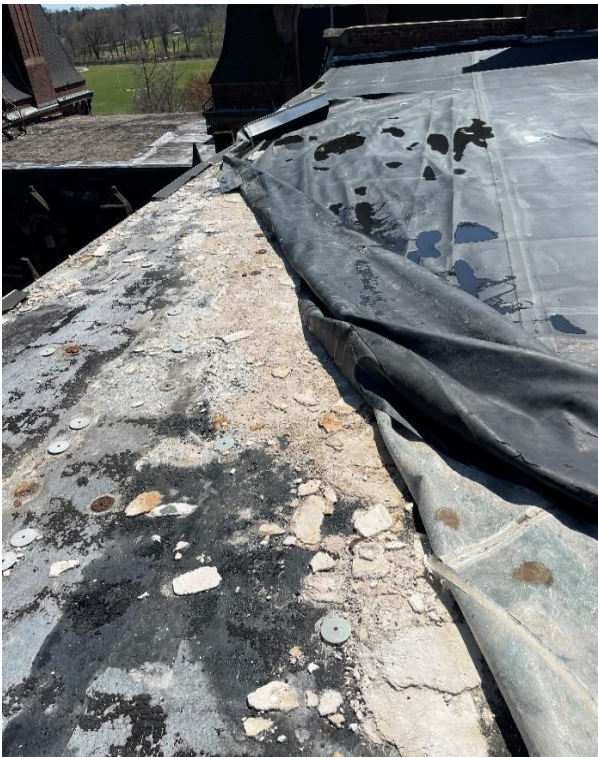
Existing EPDM roof conditions
