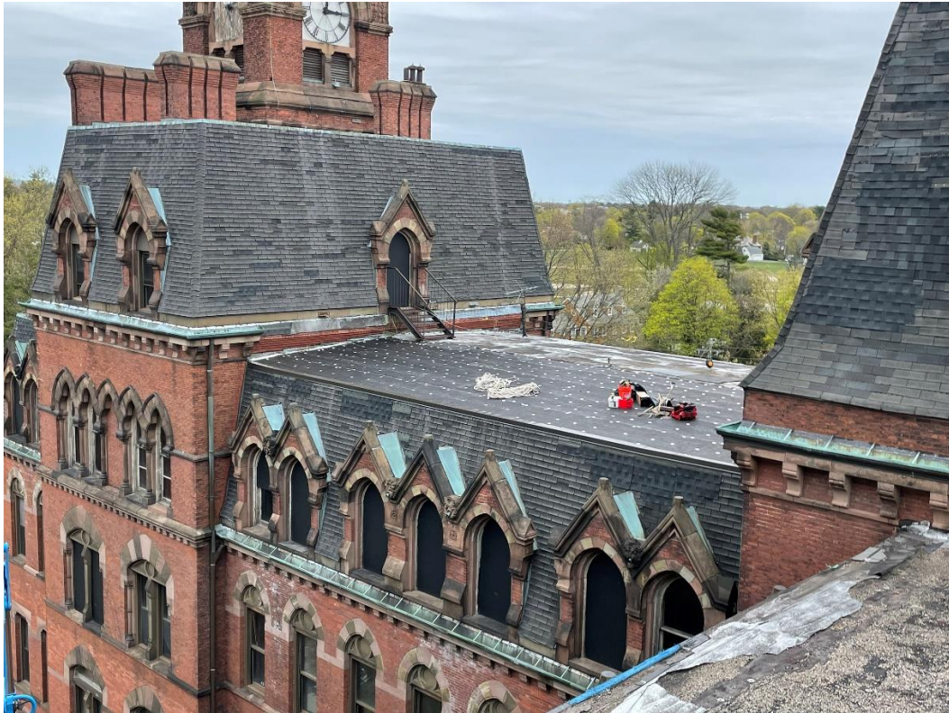
Installation of asphalt coverboard and aluminum edge flashing
