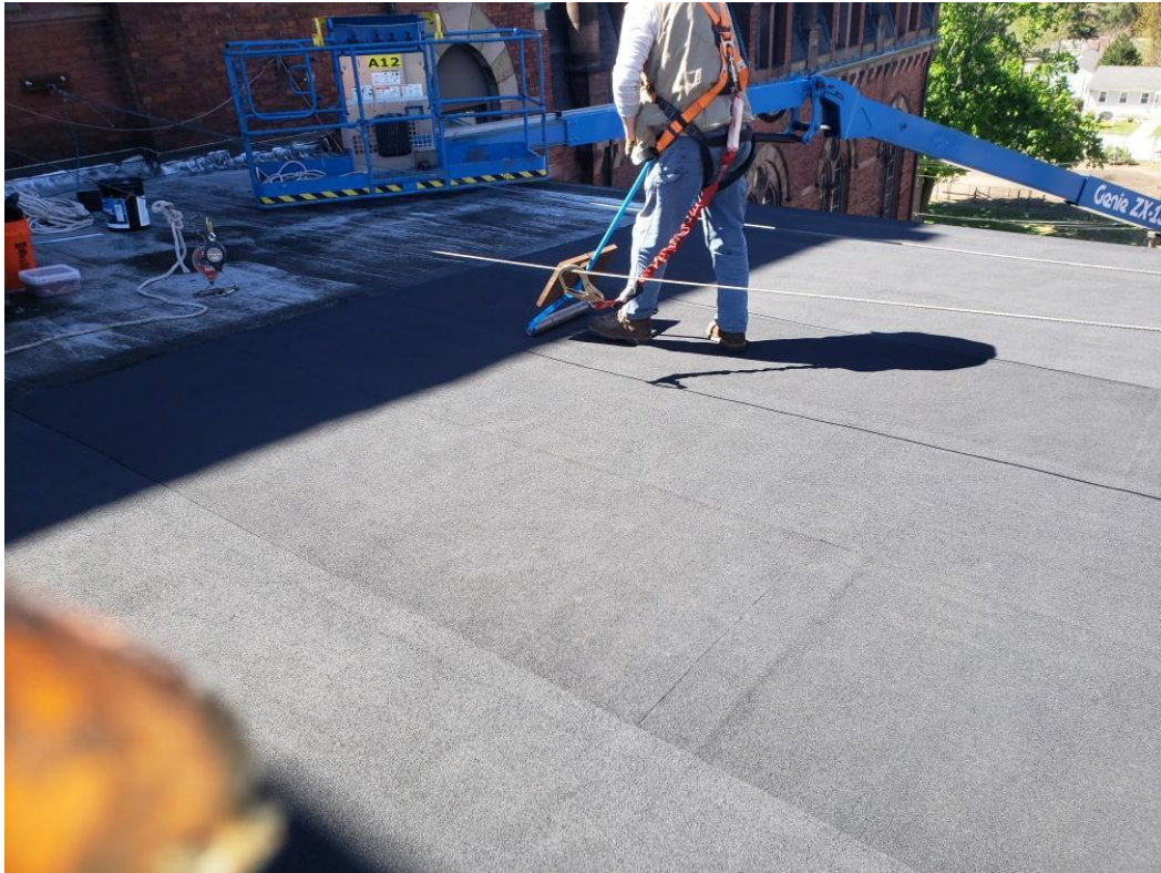
Installation of single ply, self-adhered SBS roof membrane
