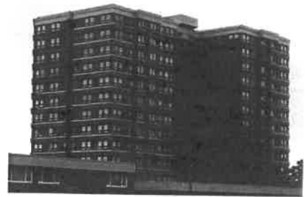
Hanover House , a residential tower block in Sheffield, with its cladding partially removed after failing fire safety tests following the Grenfell fire
