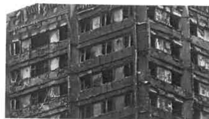
The top floors of Grenfell Tower after the fire, showing the burned insulation, with portions of the original structure revealed underneath. The cladding had melted.
