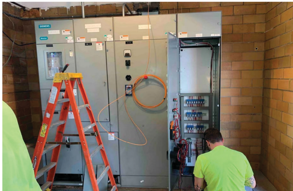
Electrical and communication panels for Well No. 10 being wired.
