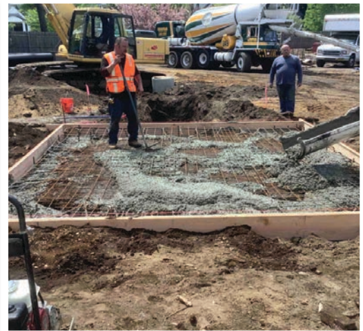
Concrete is placed for the new H2O2 tank pad for Well Nos. 8 and 12.
