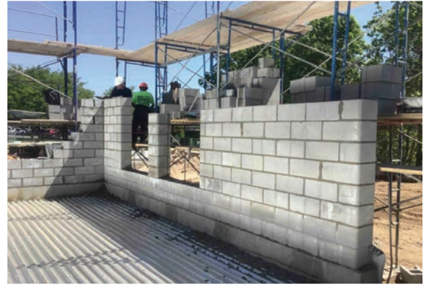
Decking for first floor and block work for Well Nos. 15 and 16.
