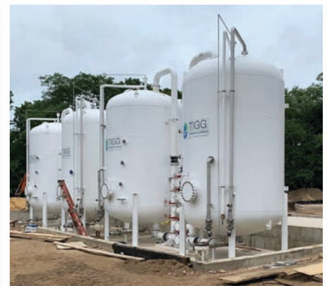
Granular Activated Carbon (GAC) filters being installed at the Clinton Road well site.
