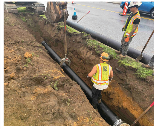
Village Water Department crews installing new water main on Cherry Valley Ave near the DPW garage.
