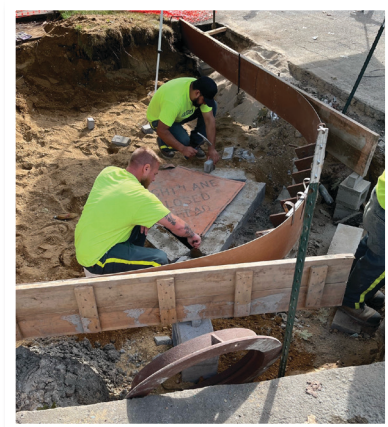
Frank Brusack and Yigael Moises Jimenez working to rebuild a Village catch basin/drywell.
