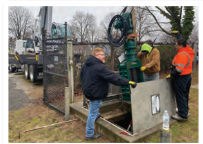
Sanitary Lift Station pump replacement
